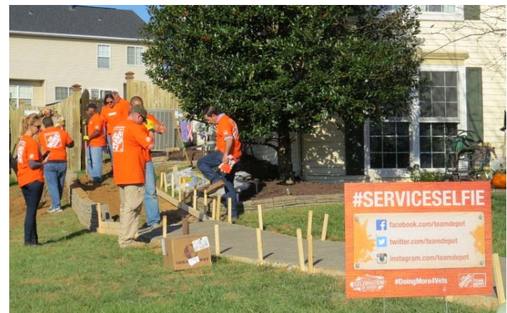
The concrete rear access ramp under construction.
