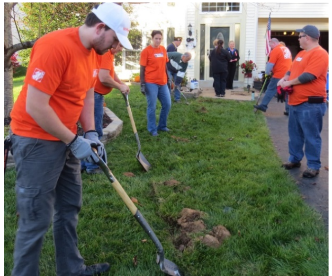
Construction of the entry ramp begins with some serious shovel work.
